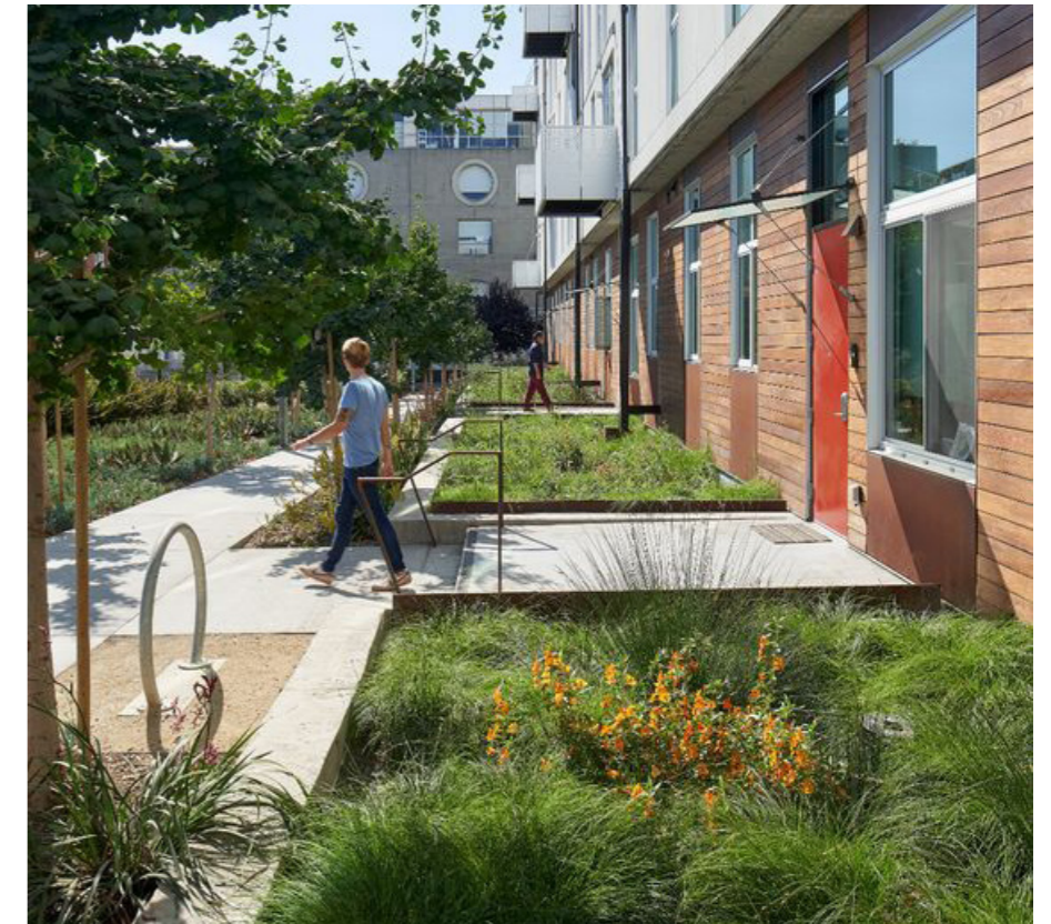
Rain gardens as part of the naturebased SuDS solutions. Reference: Brannan street, San Francisco
