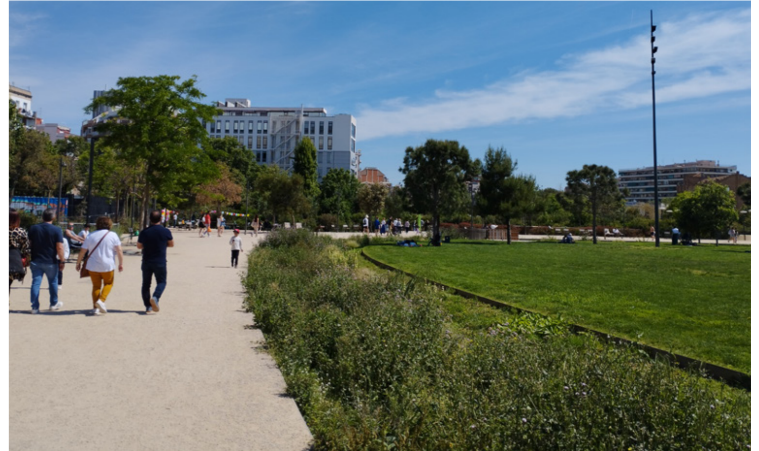
Nature based solutions for SuDS play an important role in flood prevention, water retention and detention and filtration. Reference: Plaza des les Glories Catalanes, Barcelona - Swale
