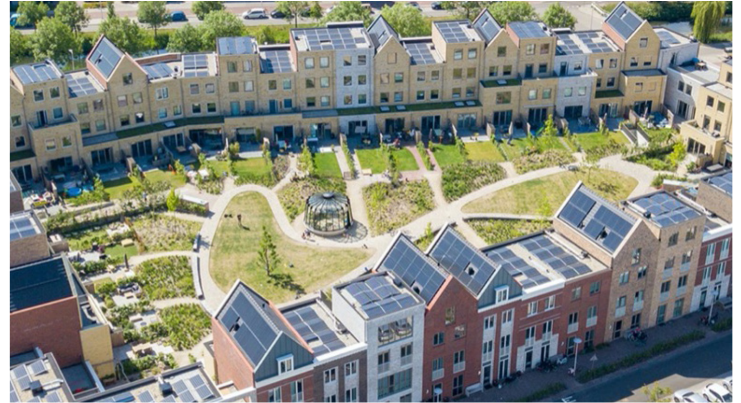
Balance between Privacy and Sociability, privacy screening (planting, swale timber panels, distance from communal shared space), but direct access to communal courtyard space from apartments
